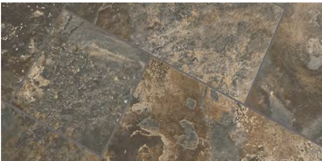
Matching the grout color to the tile results in less noticeable lines between each tile and creates a more fluid look to the floor.
